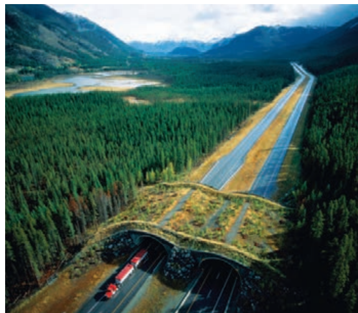
FIGURE 4.2 By providing a safe way to cross barriers such as roads and highways, land bridges such as this one in Canada allow animals to move safely from one part of their habitat to the next.
