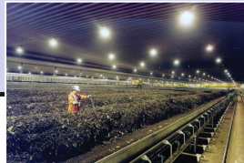
(b) Aeration building, Edmonton composting facility Copyright © 2008 Pearson Education, Inc., publishing as Pearson Benjamin Cummings
